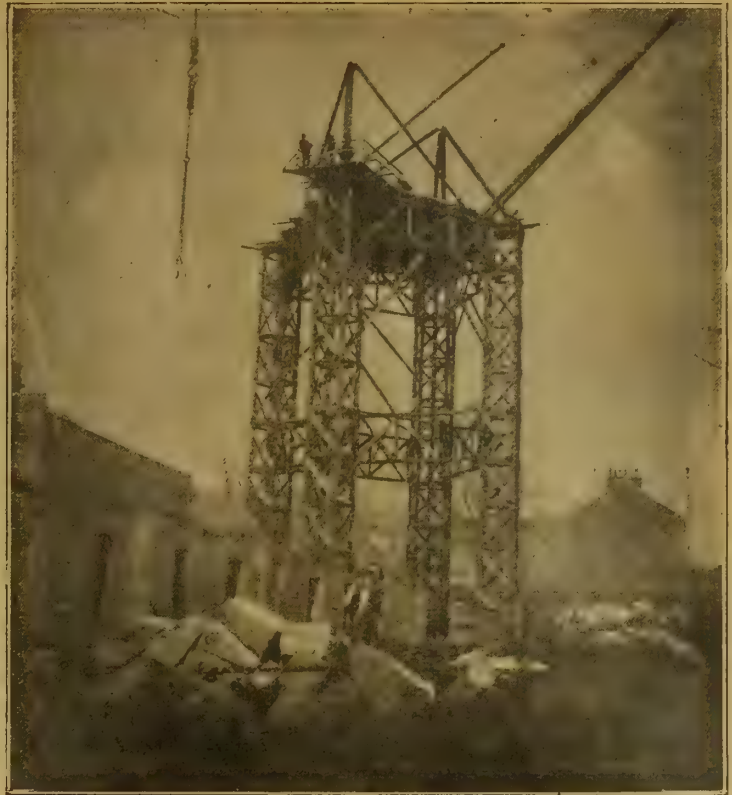
FOUR-LEGGED CRANE SCAFFOLDING.
